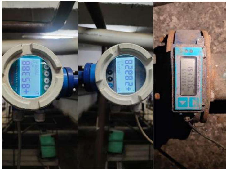
STP INLET AND OUTLET METERS
